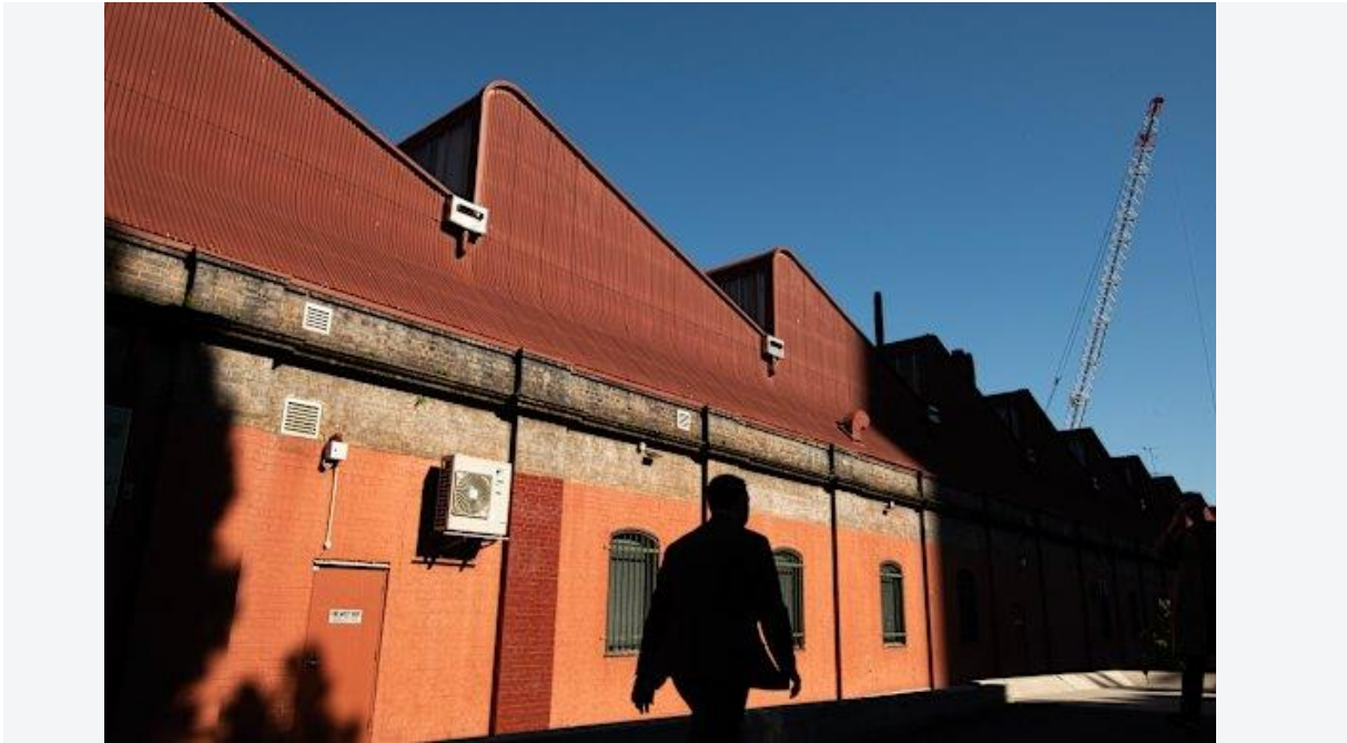
The Harwood building housing museum offices and workshops. STEVEN SIEWERT
