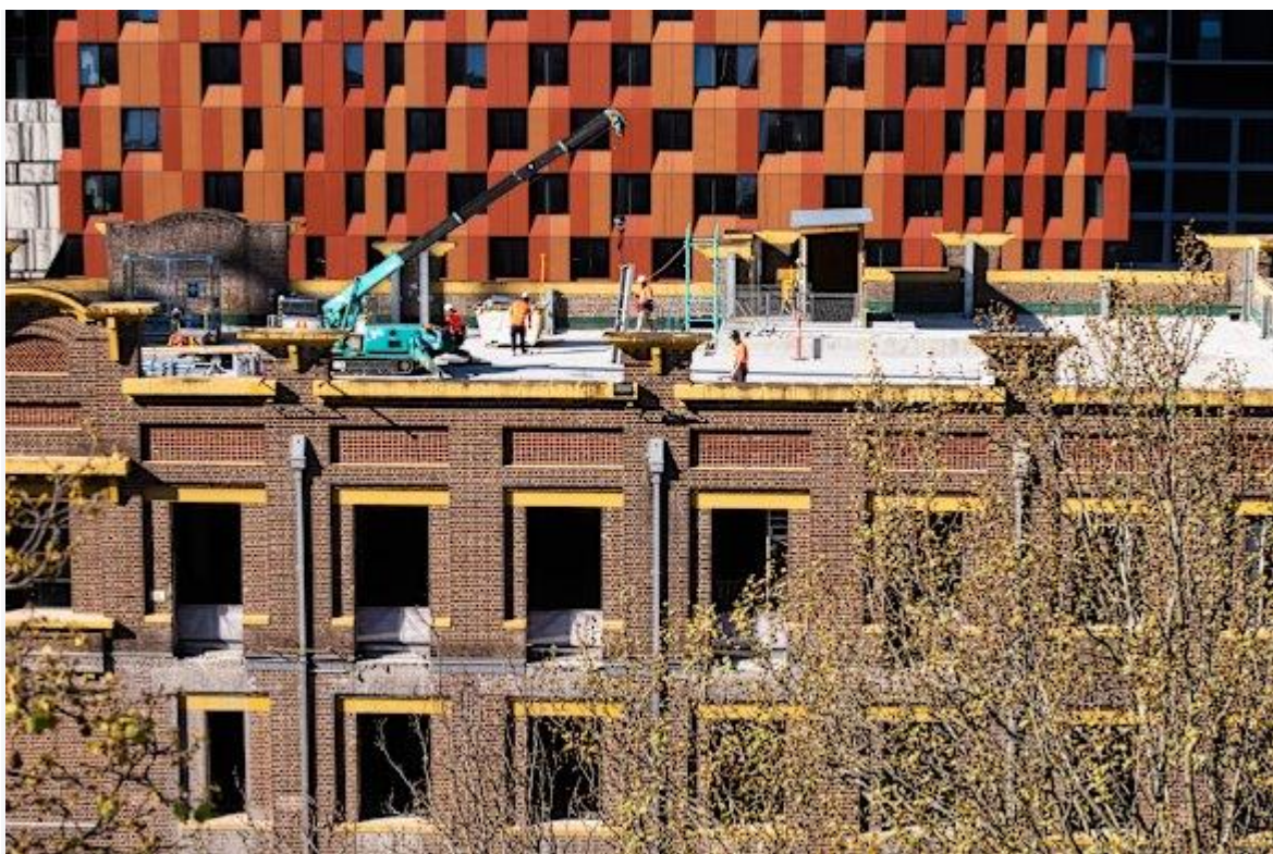
Construction on top of the Switch House at Powerhouse Ultimo. STEVEN SIEWERT
