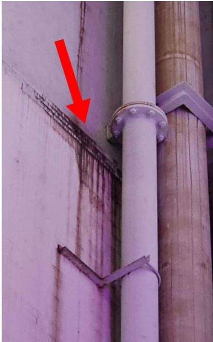
L: Significant brickwork cracking at chimney stack in Boiler House. Supplied Image R: Water leak, signs of efflorescence and water marks in Switch House north wall. Supplied Image.
